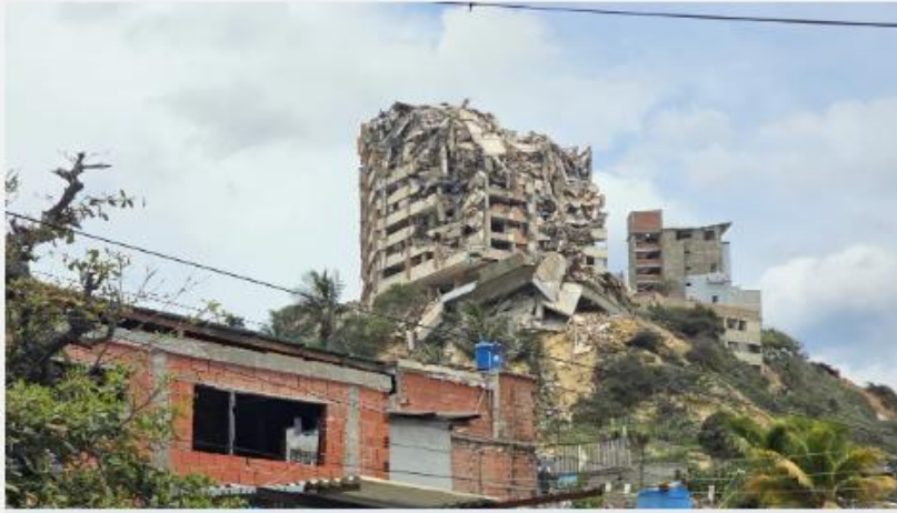
Many buildings were damaged or completely destroyed following the earthquakes. Here, buildings in La Guaira, Venezuela. Photo: LWF/María Laura Caba
